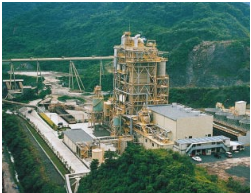
61MW CFB Power Plant for Sumitomo Osaka Cement Co., Ltd. Kochi Plant
