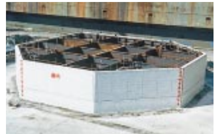
Atami Port Hybrid Caisson
