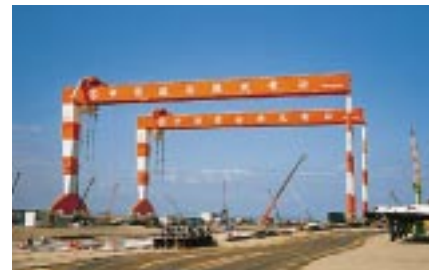
Goliath Crane for Imabari Shipbuilding Co., Ltd
